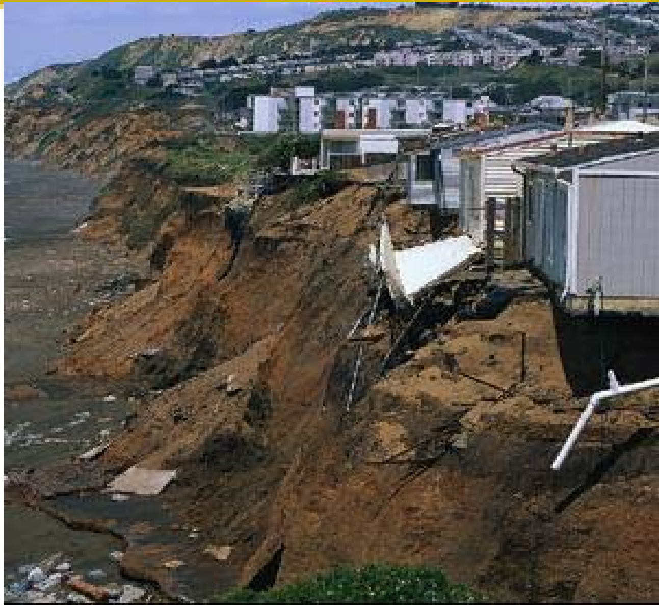
Houses undermined by coastal erosion in Pacifica, California. Photograph courtesy of NASA .
